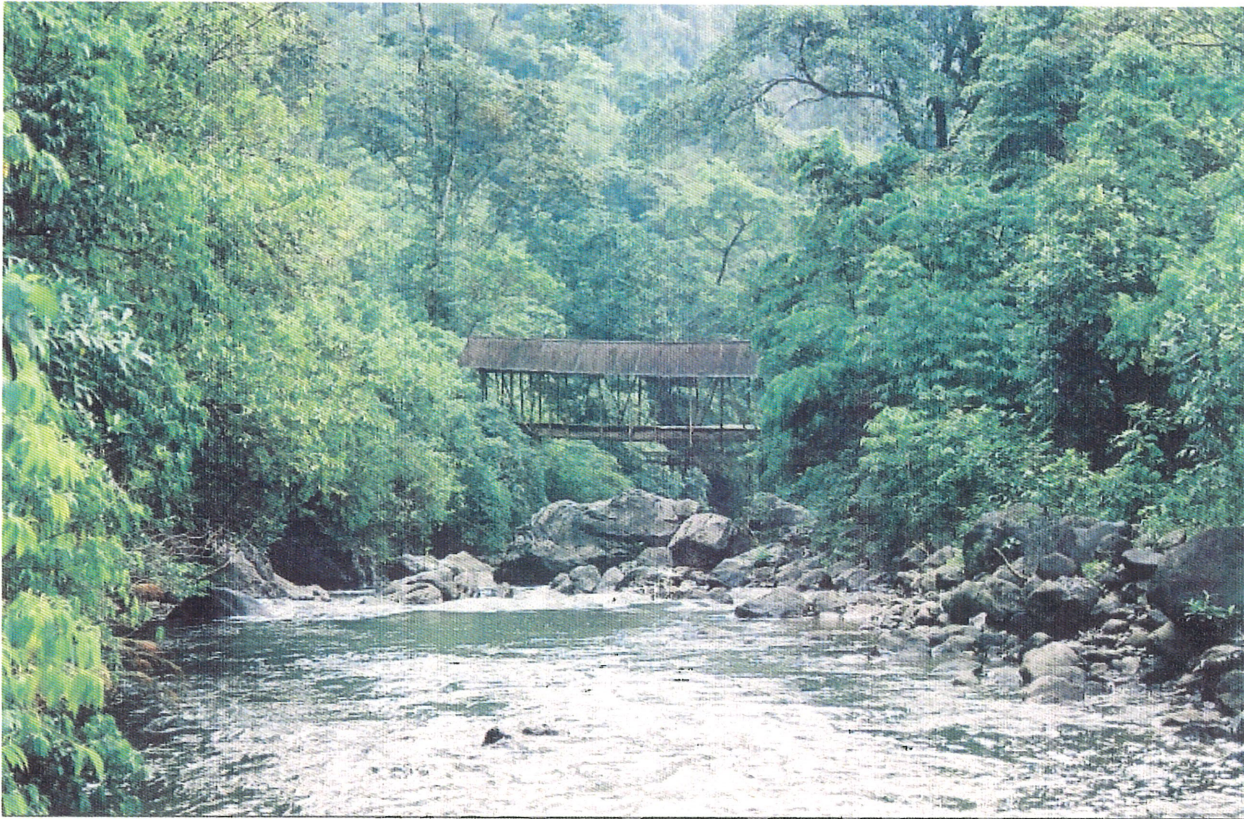
7. A view of the 70-year old wood bridge as seen from the Ecotourism Center along the Panima River.
